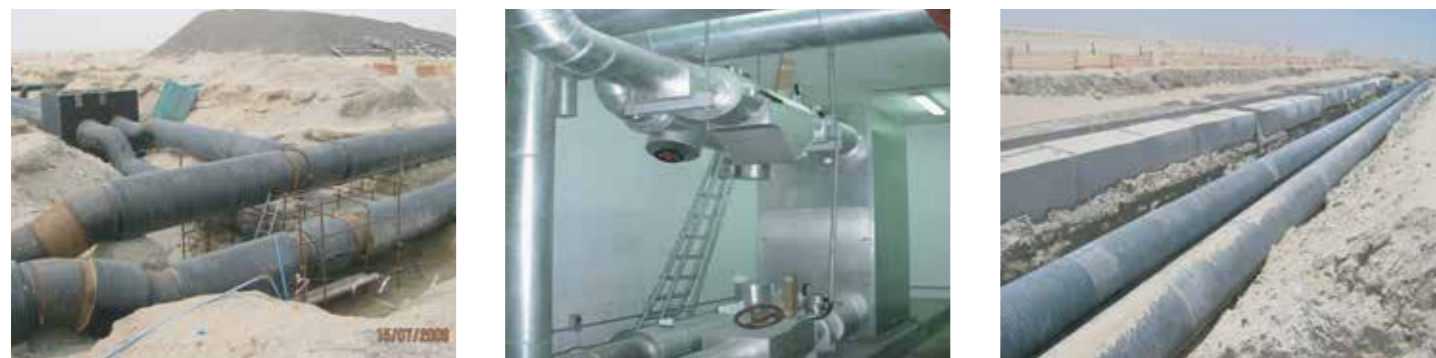
Installation Works-District Cooling Piping Network by Gargash Insafoam LLC
