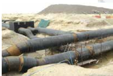
Installation Works-District Cooling Piping Network in U.A.E. Dubai
