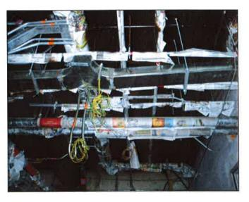
Protecting by wrapping the ceiling tee and other services with plastic cover before spray.
