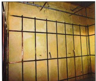
Insugard Spray Polyurethane foam is a sprayapplied insulating foam that is installed as a liquid and then expands from its original size. It can be adjusted and have many different physical properties depending on the use desired.
